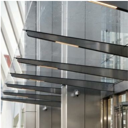
RF:01: Glass skylight to 20% of canopy to comply with Fire Safety regulations
